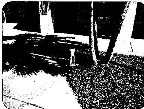
Broken sprinkler heads are a common problem encountered during irrigation evaluations at schools.
